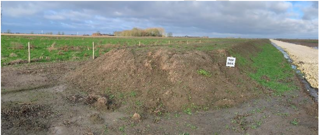
Insert 5: Temporary Topsoil Storage (January 2023)
